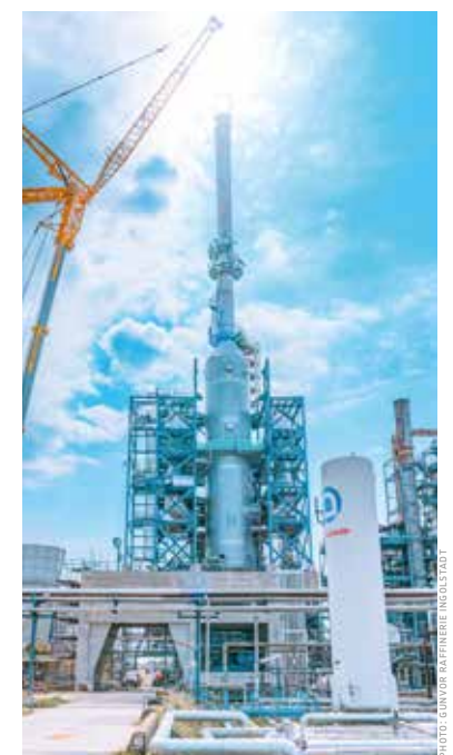
Lifting of the lower column section – diameter 5.8 meters, length 19.1 meters, weight 52 tons – onto its foundation.
