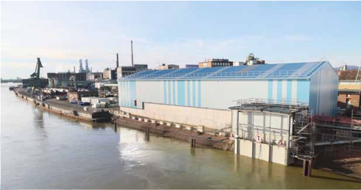
The new river water plant supplies the industrial park with 15,000 cubic meters of water per hour.
