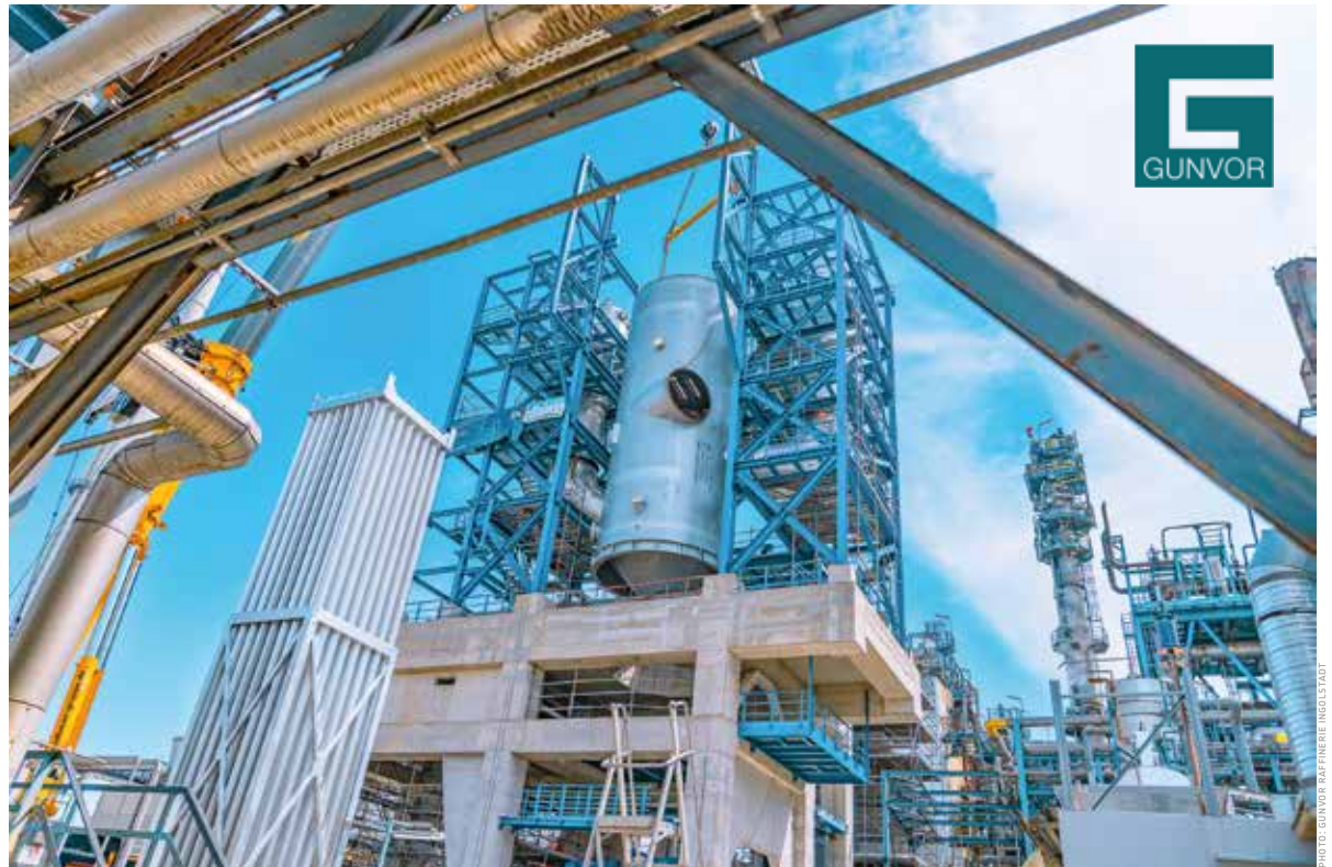
Lifting of the lower column section – diameter 5.8 meters, length 19.1 meters, weight 52 tons – onto its foundation.
