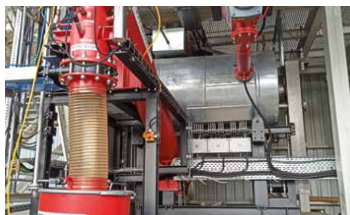
▲ ► The new pilot plant of Fraunhofer IKTS.
