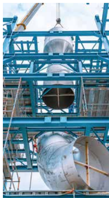
Lifting of the lower column section – diameter 5.8 meters, length 19.1 meters, weight 52 tons – onto its foundation.
