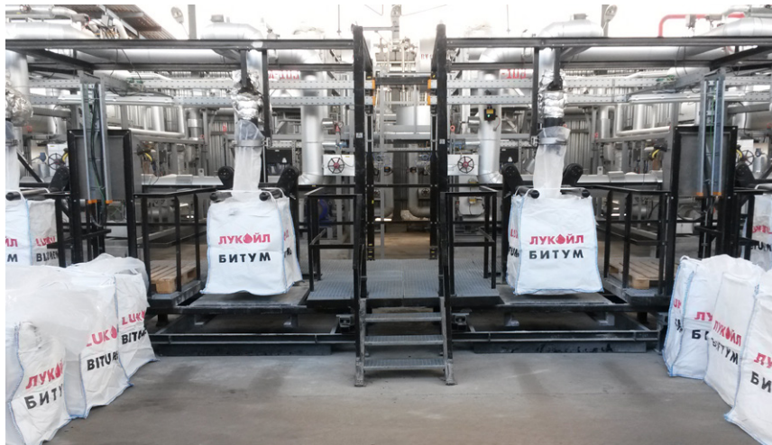
Bitumen Cooling and Packing Unit at LUKOIL Refinery, Russia
